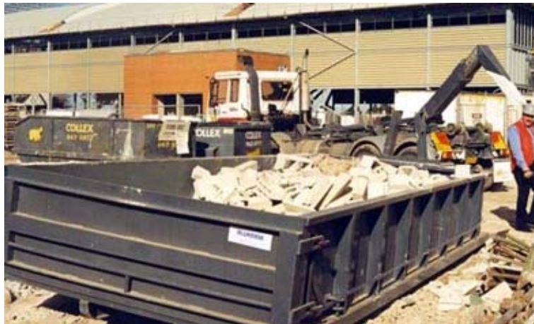
Larger sites have capacity for multiple bins, maximising the opportunity for source separation.
