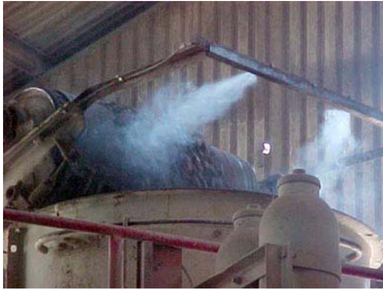
Mist sprays at conveyor transfer points are an effective way of minimising dust emissions
